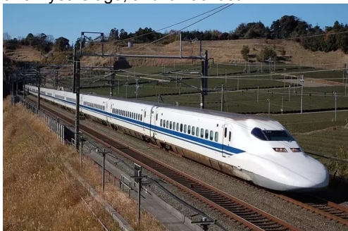
In October 1964, Japan launched the Shinkansen High-speed Train Service. Sometimes better known as "bullet trains", these high-speed trains initially ran at 210 km/h. With new rolling stock and improved technology, they now run at 320 km/h on some sections.
